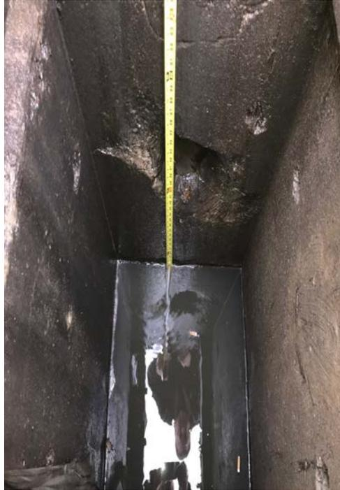
Photo 1 – Catch basin after a winter of treated salt usage on area roads. The sump remains empty of debris and only melt water is left.
